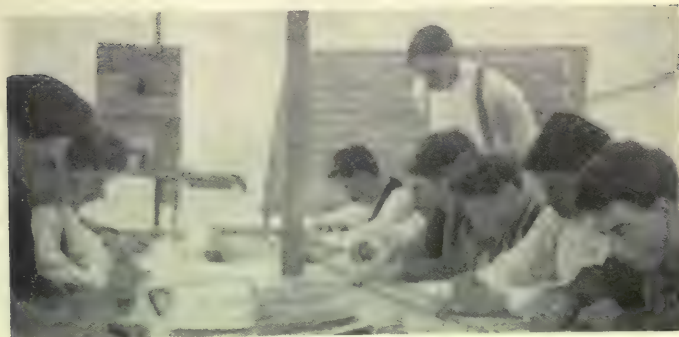
Frontier College on Railway Construction. Instructor C. O. Banting teaching his fellow-navvies. Southern Saskatchewan, 1909.
